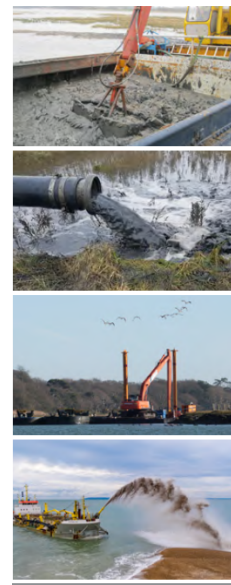
Figure 2.2: Different disposal techniques, from top: Clamshell excavation from hopper (Cefas/Reda); release of hydraulically pumped sediment via pipeline (Eco Environmental Ltd.); spit barge and hopper barge at marsh transfer and hydraulic pumping station (ABPmer); and coarse sediment rainbow discharge (Boskalis).
